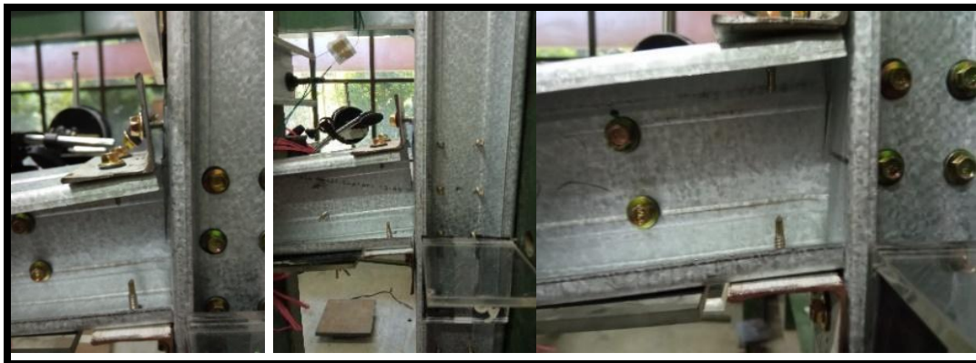
Figure 4.11. Failure at the Angle cleats-Screw Joint
