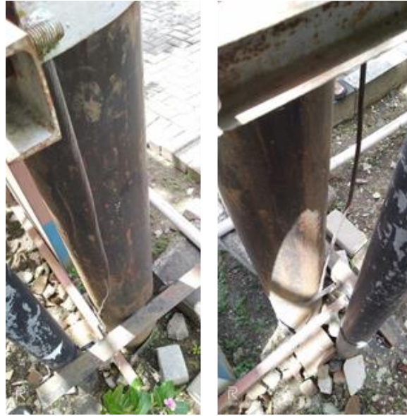
Gambar 4. Kabel Pentanahan
